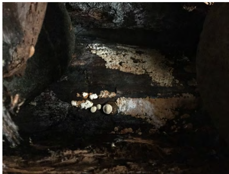
Top layer of stringers
