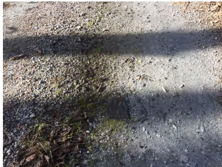
Running directly on stringer
