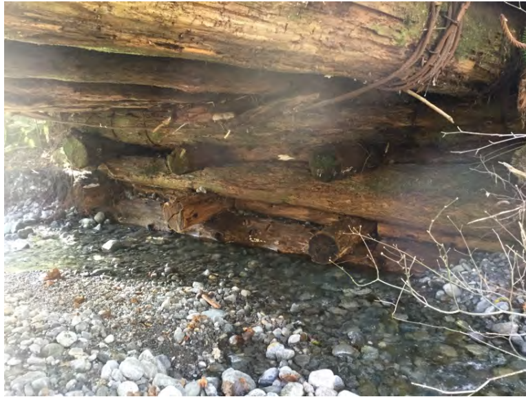
Right Bank Abutment when facing downstream
