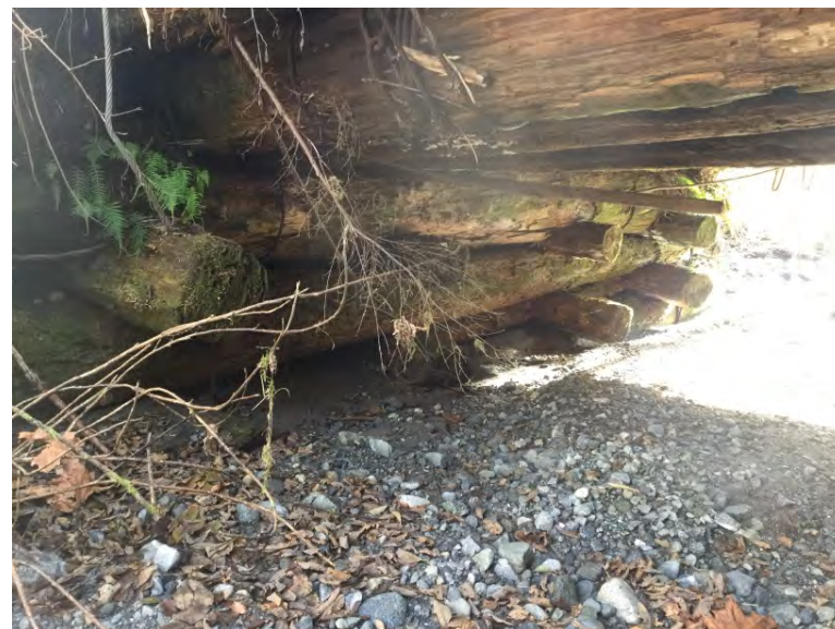
Left Bank Abutment when facing downstream
